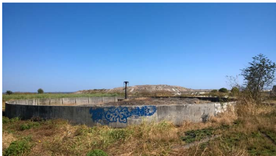
Copperbelt Province – Chingola – Old Trickling Filter at Ponds Site
